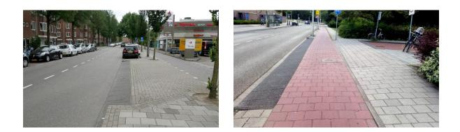
These entrance kerbs are arranged in a straight line as a continuation of the ordinary kerbs on the main carriageway, without any indentation which could suggest the beginning of a side road. In addition to specifying the use of entrance kerbs as a defining feature of an "exit", Dutch guidance also specifies that there must not be any kerb corners which might imply the beginning of a section of carriageway.
