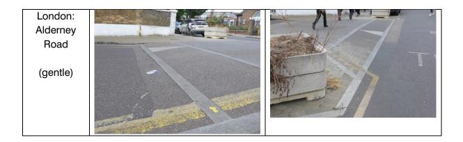
Note that other factors, beyond actual ramp design, also affect how easily a ramp is driven over. These factors include the degree of crossfall on the footway and on the carriageway, and any incline along the side road (as visible at Woodside Avenue and Scott Street in the images above).
