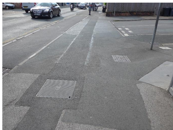
Looking toward junction (pedestrian's view)
