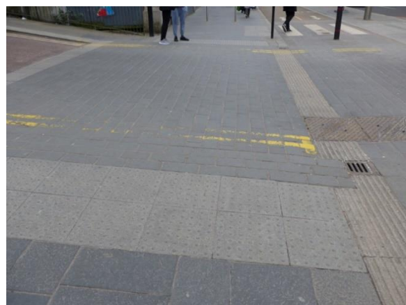
Tactile paving detail (looking toward side road)
